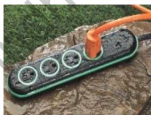
Fig: 15.24 Electrical extension placed damped environment
