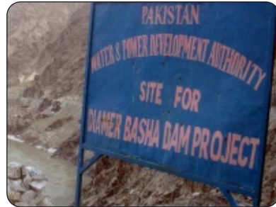
View of Under Construction Diamer Bhasha Dam
