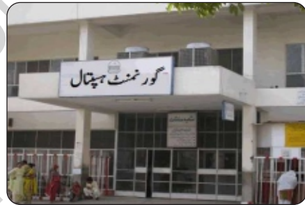
View of a Govt. Hospital
