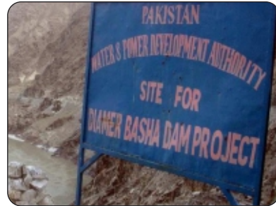
View of Under Construction Diamer Bhasha Dam
