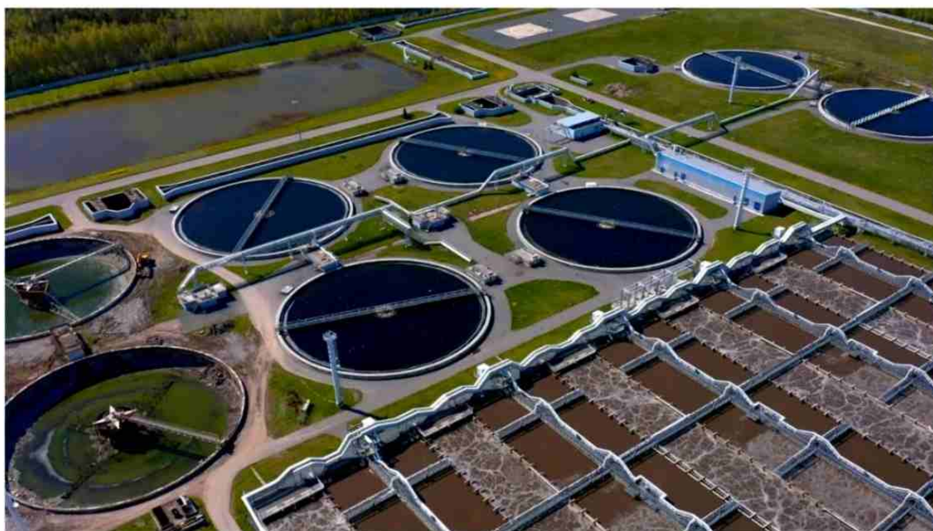
Fig. 27.7 Sewage treatment plant
