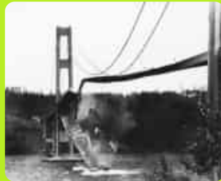
The collapsed, Tacoma Narrows Bridge.
