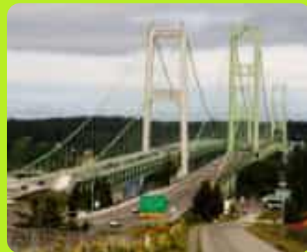
The newly built Tacoma Narrows bridges opened in 1950 (right) and 2007 (left). These bridges are built with much higher resonant frequencies.
