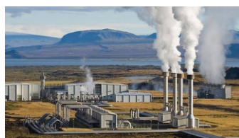
Fig 8.11(b) Geothermal power plant
