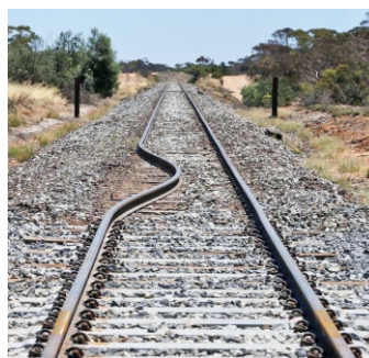
Fig 9.7 (a) Thermal expansion
